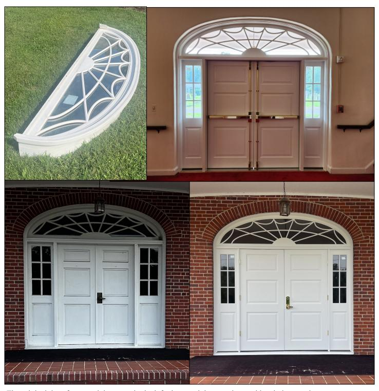
The original door frame and doors are in the left photo and the new doors, side windows and transom are on the right. The doors are now the proper size for code and they also swing outward, rather than inward, which is also required by code. The inside of the door is shown in the top right photo. Thanks to all who helped support this project through your financial gifts.
